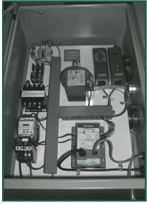
■Advanced electrical controls include an airflow switch and temperature stat, and allow field selecting either 230V or 115V power.
