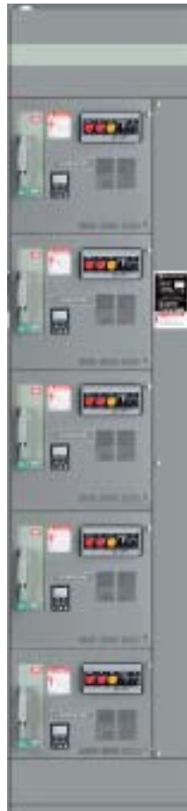
8998 ATV58 MCC Panel Section.tif
